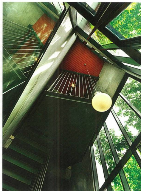
THE SUSPENDED STEEL STAIRCASE THAT GOES UP TO THE FIRST AND SECOND FLOORS OF THE HOUSE. DR TAN USED STEEL BECAUSE IT IS SO PLENTIFUL IN THE COUNTRY.
