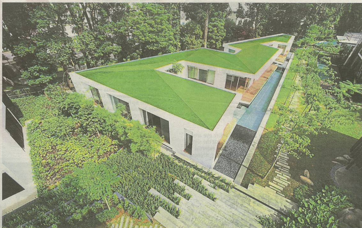
Zig Zag House, Singapore: Set on a triangular site, the house twists around a mature tree located on its premises, creating courtyard spaces that are sheltered from the harsh weather but allow for light and cross ventilation into the interior and basement level. Internal corridors serve as breezeways between air-conditioned and naturally cooled areas. Slightly lofted above the ground, each of the building's three wings houses an entertainment zone, a family zone and a private master zone. Unfortunately, during construction, the tree roots were damaged and a new tree had to be planted. — Photos from Ministry of Design
