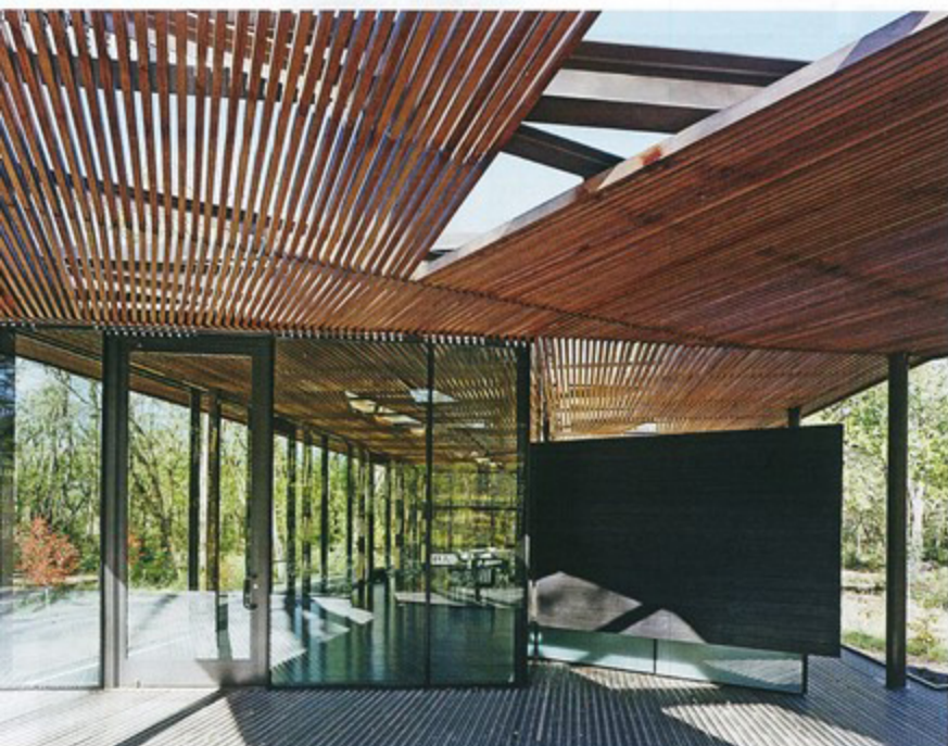
The Visitors Pavilion at the Indianapolis Museum of Art in the US, designed by Marlon Blackwell Architects
