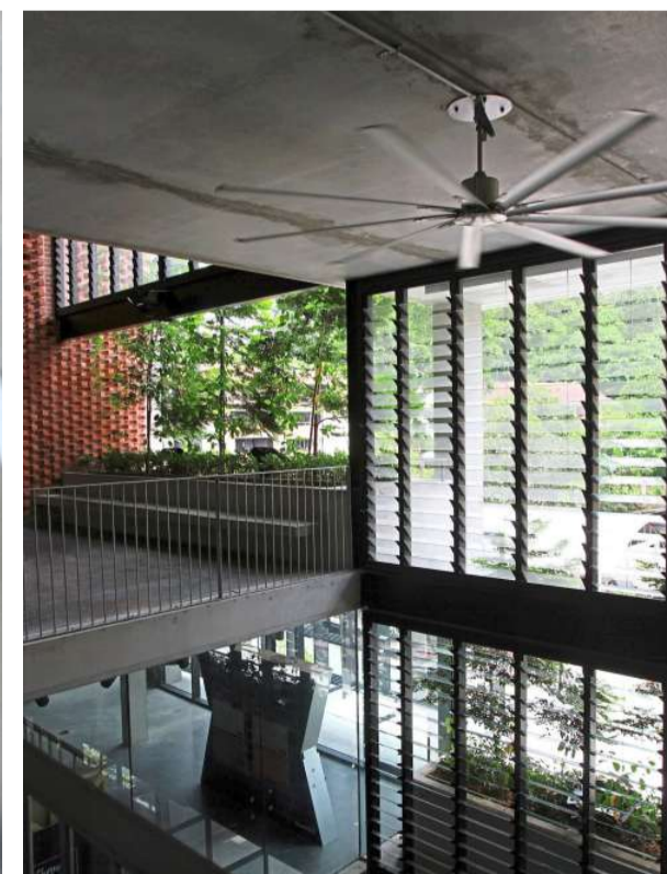
Large numbers of louvres afford good control of light and shade and air flow.
