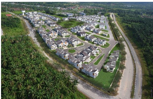
Figure 2 Honeycomb Housing at Bernam Jaya
